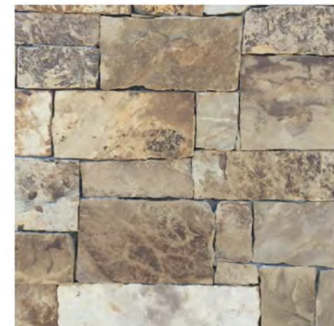
B. STONE VENEER, KO NATURAL STONE - SIG- NATURE COLLECTION MULTI, DRY STACK
